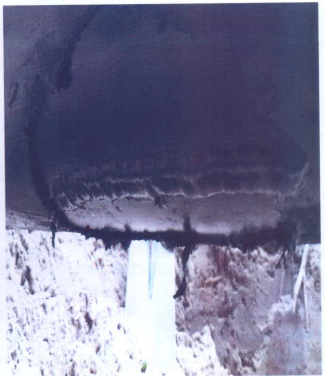
INCIDENT POINT DURING EXCAVATION
